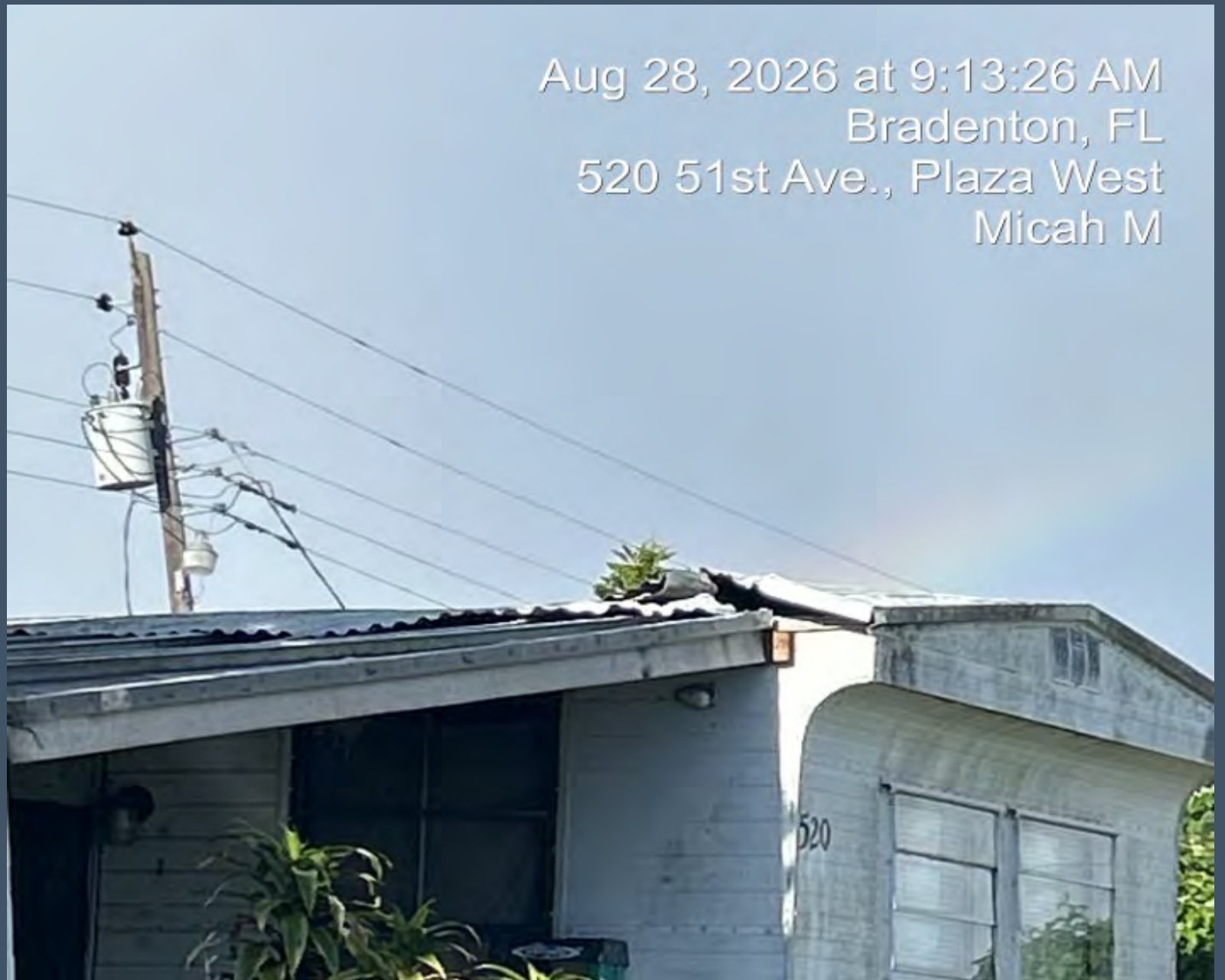
Current Photo of Roof
